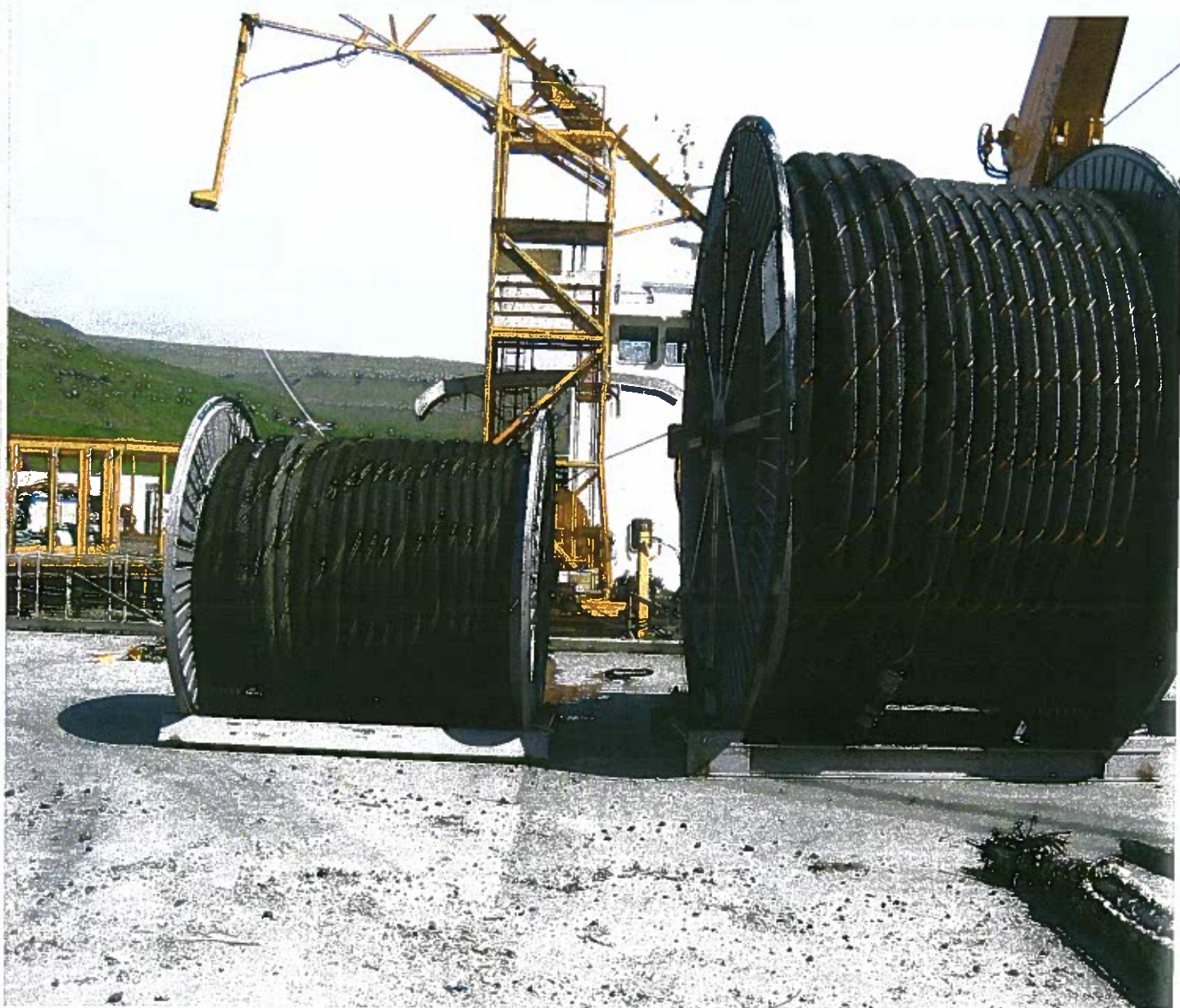
DRUMS WITH 20 AND 60 KV SEA CABLE
