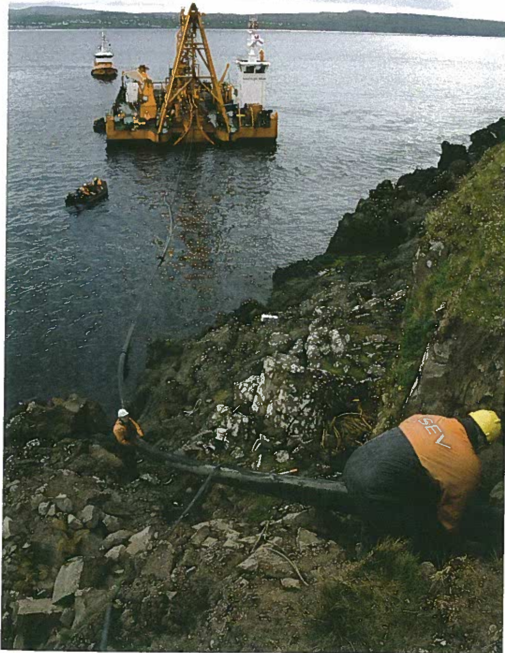
THE CABLE VESSEL NAUTILUS MAXI, THE 60KV SEA CABLE IS TAKEN ASHORE
