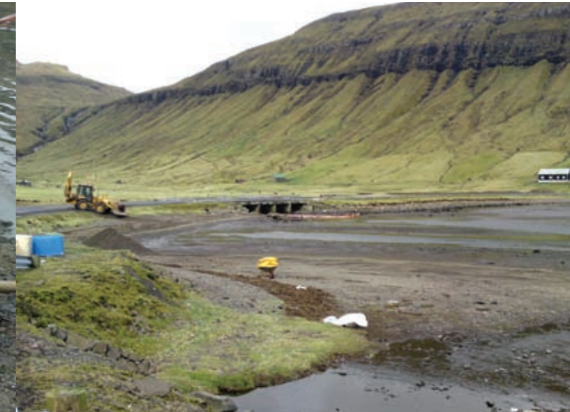
Photo 2: Bark was spread over the oil, and then the oil-contaminated sand and bark were dug up and disposed of.
