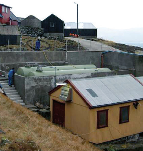
The new tanks in Skúvoy have now been installed. Foto: Hans Jákup Petersen.
