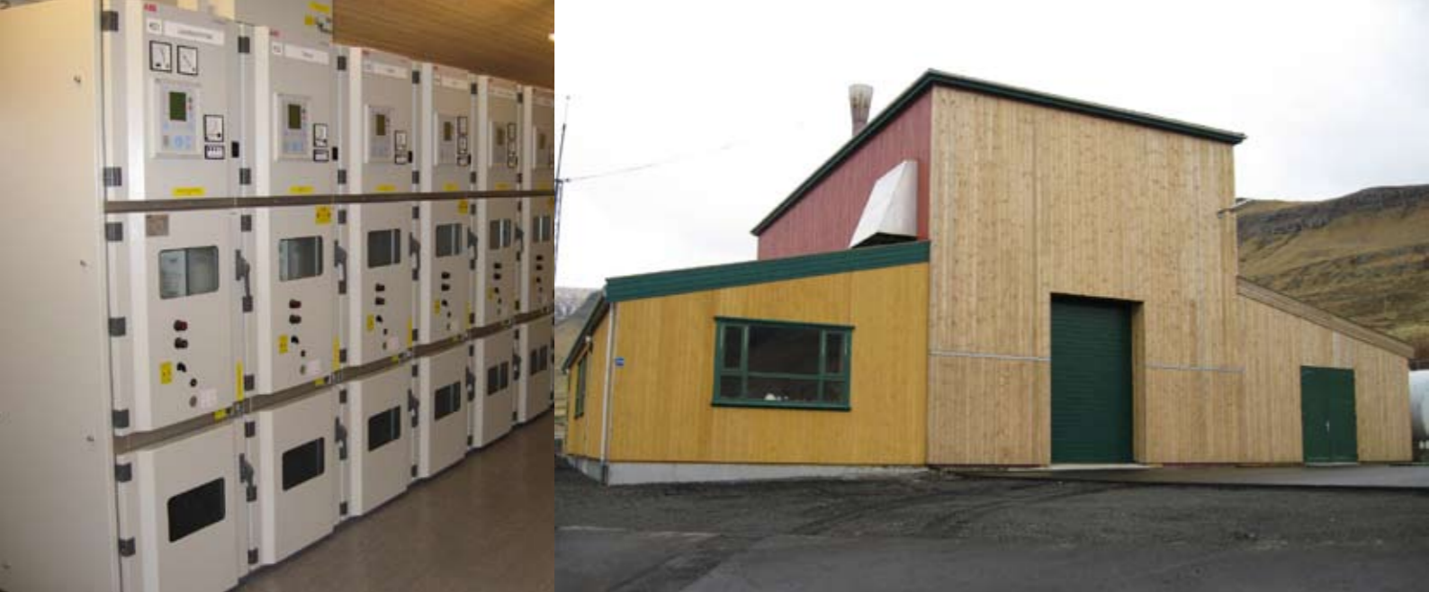
Inside the new substation.
