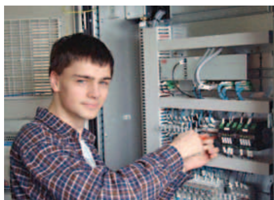
Sjúrður Samuelsen is installing the control system of the new magnetisation equipment for Generator 1 at the Fossá Plant
