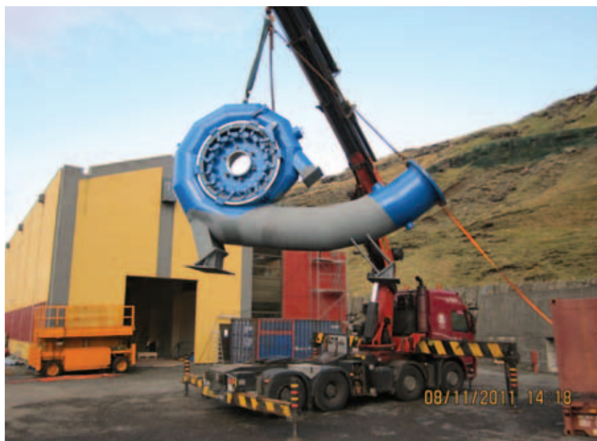
Valve and turbine 3 hoisted into place
