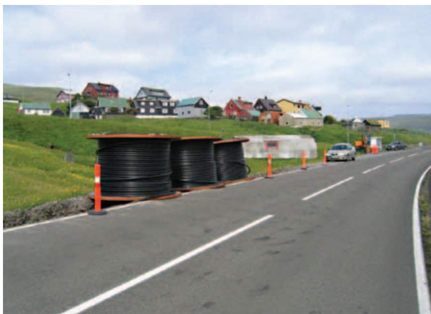
Overhead lines replaced by underground cables
