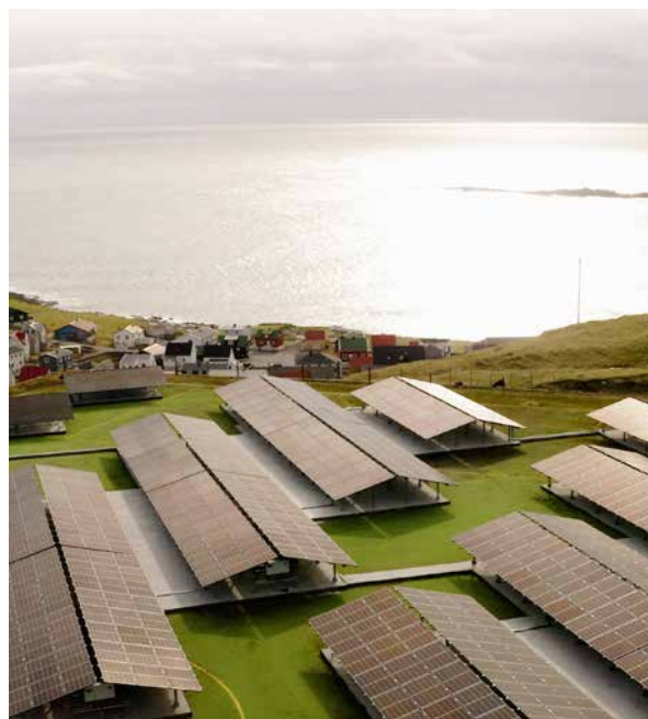
Sumba solar power plant
