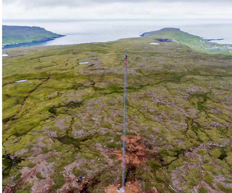
Wind measurement tower in Porkeri
